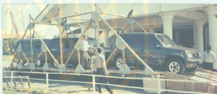
Gambar 2. 50. Sistem sambungan bambu morisco (sumber: www.moriscobamboo.com )
